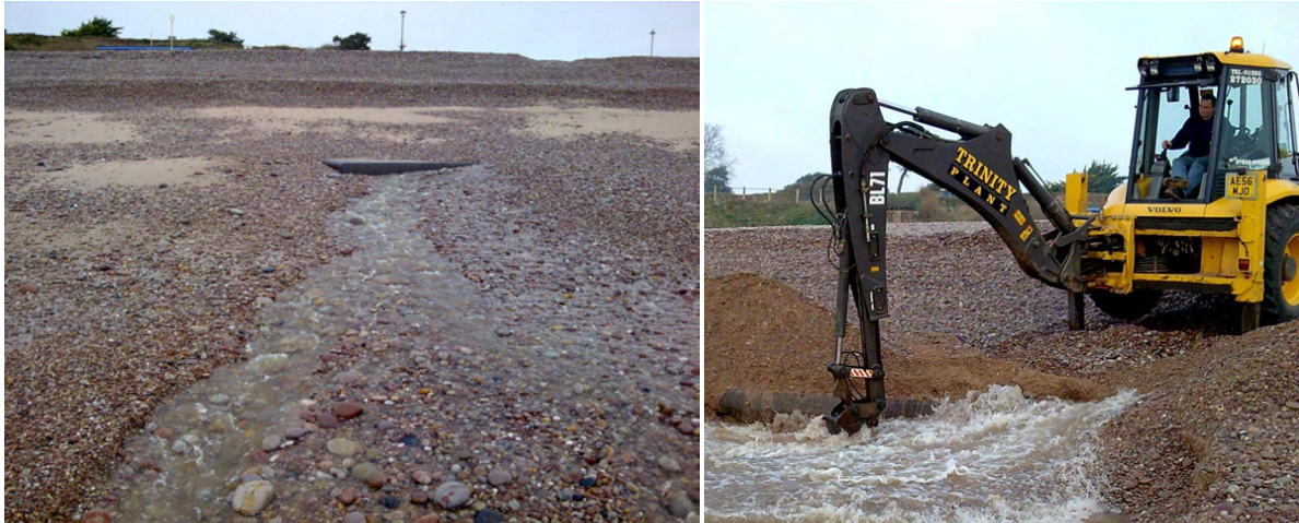
Figure 12: Photographs of the embanked compartment outfall on the pebble beach locally to the Lime Kiln, Budleigh Salterton. The left image shows the outflow blocked by gravel and pebbles. The right image shows the Council clearing the outflow which can occur weekly based on BSCC information.
